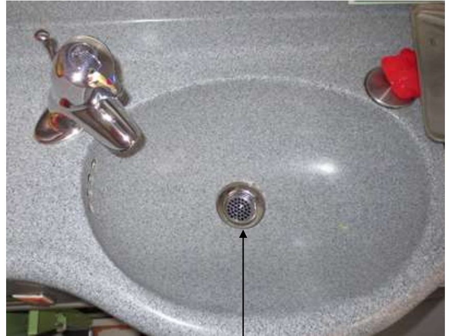
HYBRID Drain with “internal” draining
